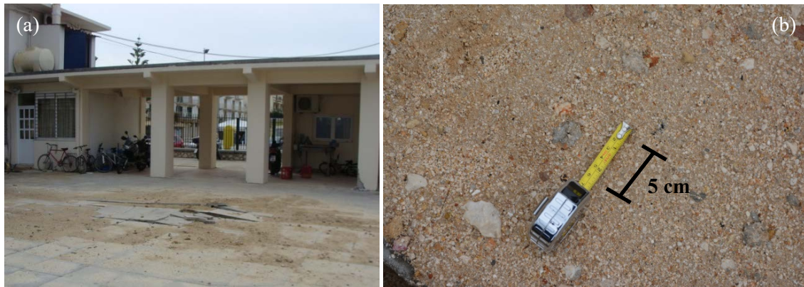
Figure 2: (a) Evidence of gravelly soil liquefaction outside the customs building of the Port Authority of Argostoli following the second earthquake ( 38.17998^{\circ} , 20.48996^{\circ} ); (b) close-up view of liquefaction ejecta on top of concrete slab ( 38^{\circ}10'47.85''\text{N} , 20^{\circ}29'24.42''\text{E} ).
