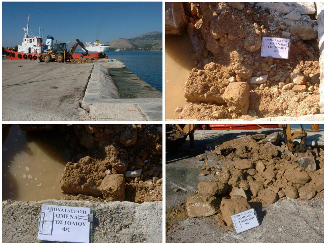
Fig. 14. View of test pit TP-1 operations and excavated material in Argostoli port.
