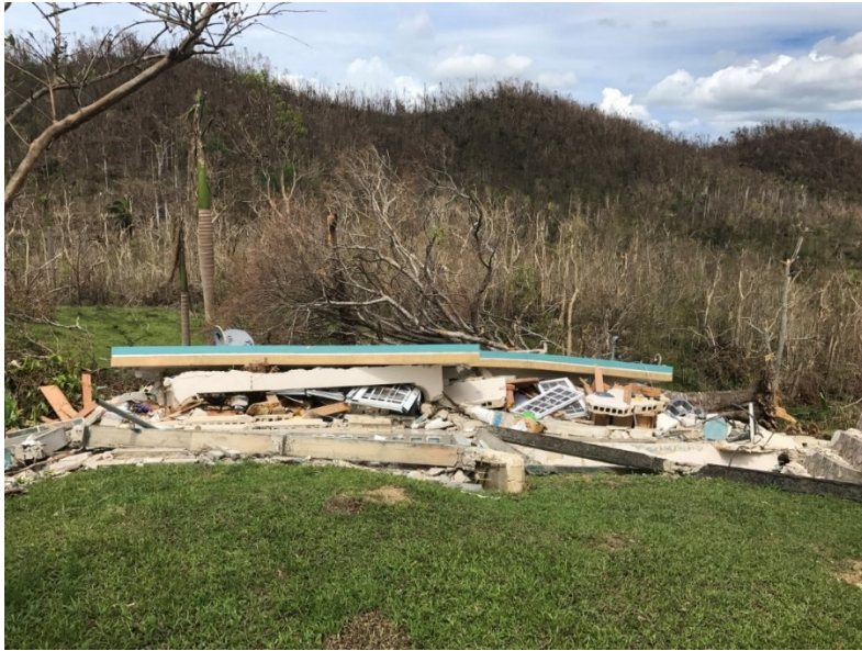
Figure 7: In some parts of the island, winds from Hurricane María destroyed concrete structures entirely.
