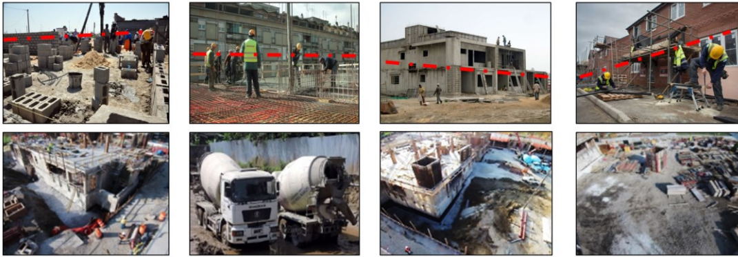
Figure 6: Absence of a horizon line in aerial visual data (bottom) obtained from construction sites.
