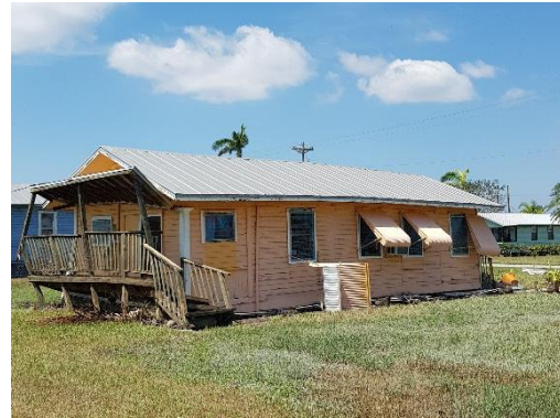
Figure 1b: Storm surge damaged house toppled off its piers in Everglades City, FL.
