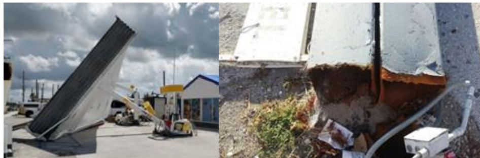
Figure 5: Damage to gas stations
