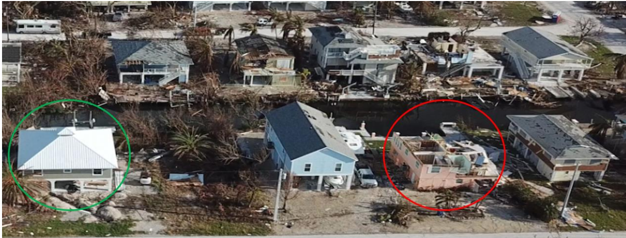
Figure 4: UAV image shows damage to low-rise houses along two streets of Ramrod Key. The green circle marks a new construction while the red circle shows an older construction.
