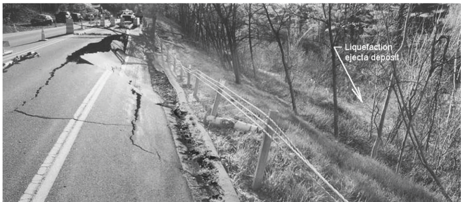
Figure 4. Road embankment failure during the M 5.0 Au Sable Forks earthquake in New York. The slide is attributed to liquefaction occurring in the fill material at the toe of the embankment. (Gingery 2003).
