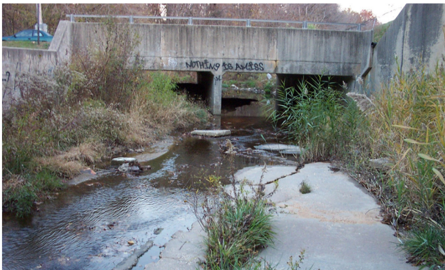
Fig. 13. (a) An in-channel bar upstream of a culvert and (b) vegetated in-channel bars on top of a fully concrete channel. (Photos by A.J. Miller).
