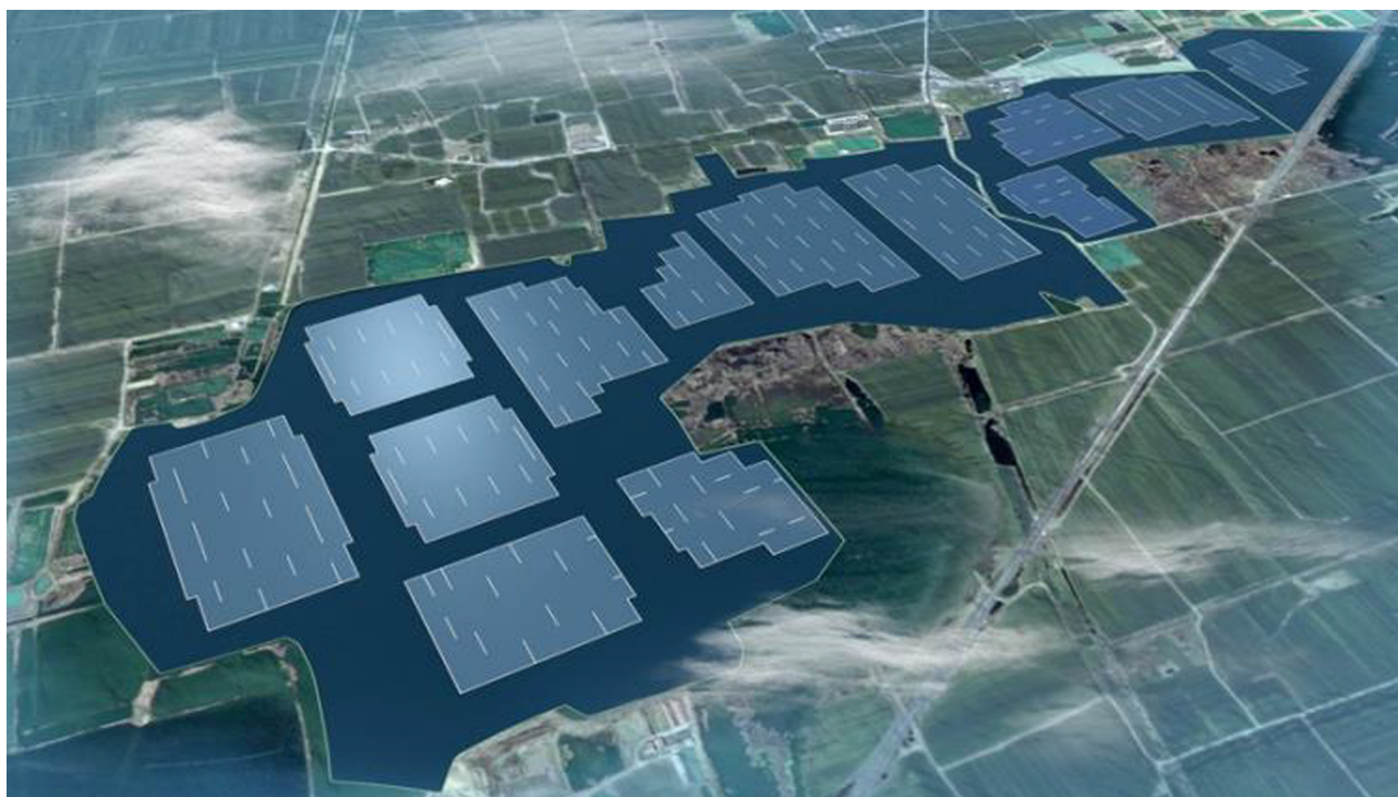
Fig. 2. 70 MW Floating PV plant on a clay quarry lake in Anhui Province, China under construction by Ciel & Terre. source: Ciel & Terre.
