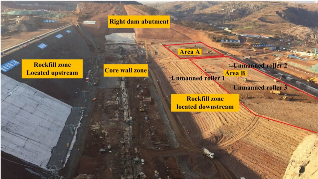
Fig. 8. Photograph of the URC system testing at the rockfill zone.
