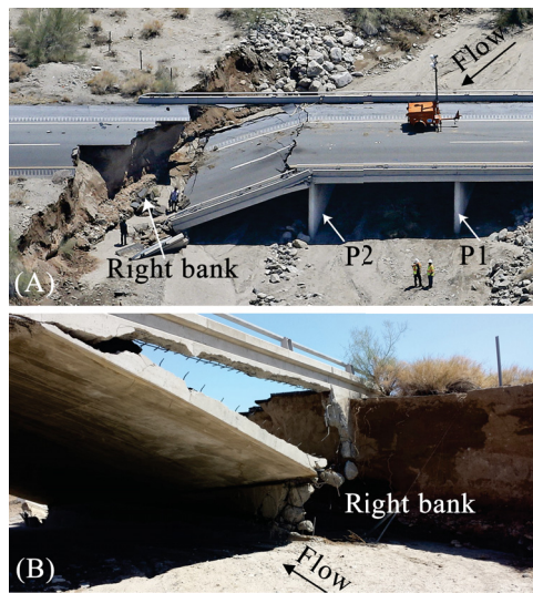
Figure 1: Pictures of the Tex Wash Bridge taken two days after the collapse of the bridge. Note the excessive erosion at the base of the right bank of the wash. (A) views upstream of the wash and shows the bridge piers herein denoted as "P1" and "P2". (B) is taken immediately upstream of the bridge piers, views downstream of the wash, and is focused on the collapsed right bank adjacent to the bridge pier "P2".
