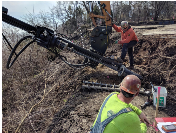
Fig. 2. Installation of screw piles (helical anchors) to be used as tiebacks in a slope stabilization project
