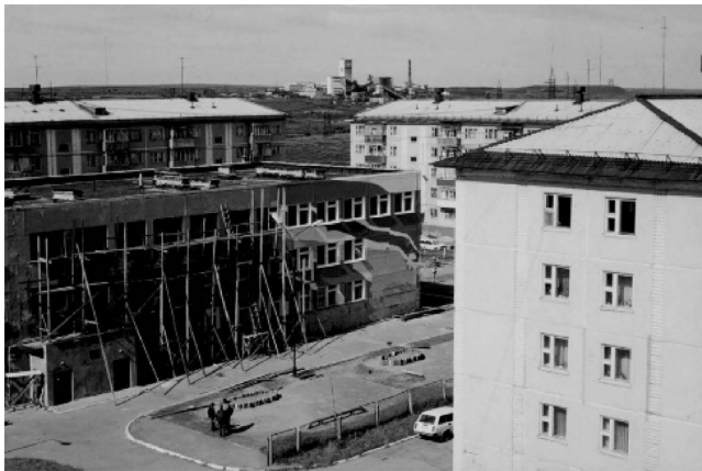
Fig. 2. Examples of prefabricated buildings in Vorkuta. Source: Britannica, Deviant Art.
