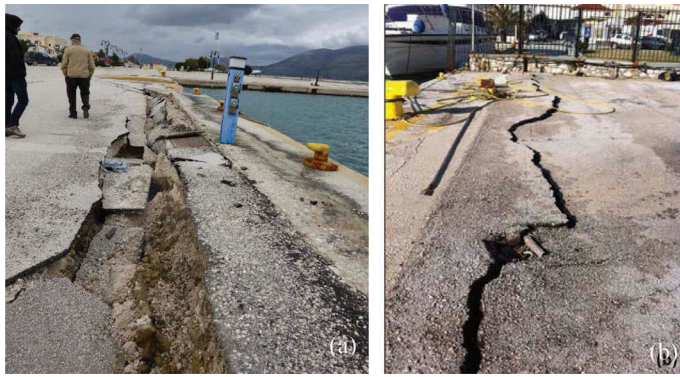
Figure 3. (a) Displacement of the quay wall in Lixouri port, across the Plaza of National Resistance following the second earthquake (GPS coordinates: 38.199444, 20.439444); (b) displacement (~16 cm) of the quay wall in Argostoli port.
