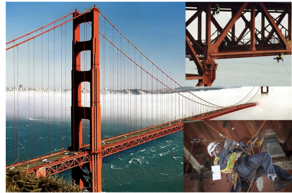
Fig. 1: Current practice of steel bridge inspection: rope certified bridge engineers inspecting the Golden Gate bridge, San Francisco, California [3], source: NBC April 2018.
