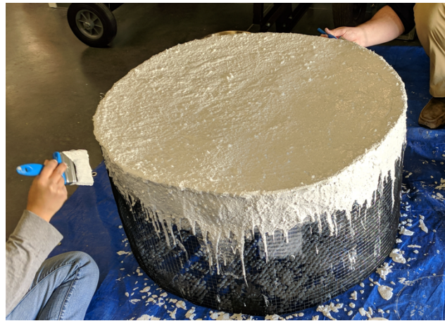
Figure 1- Building the acrylic concrete rainwater harvesting tank at the construction workshop phase of the project.
