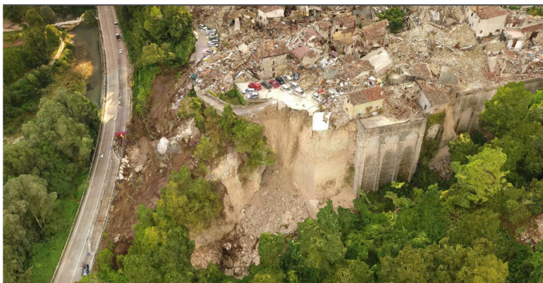
Figure 4. 3D SfM model of a slope failure in Pescara del Tronto possibly caused by a retaining wall collapse ( 42.75109^{\circ} N 13.27208^{\circ} E; SfM by Franke et al. presented in Zimmaro and Stewart 2016).
