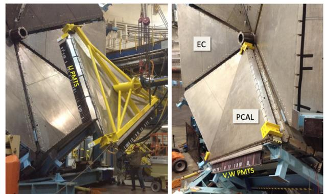
Fig. 16. Left: Installation of PCAL module onto the Forward Carriage in Hall B at the Sector 5 position. U PMTs fit into the gap between the EC modules. Right: PCAL module installed in front of the existing Sector 5 EC module. The yellow lifting fixtures were later removed. (For interpretation of the references to colour in this figure legend, the reader is referred to the web version of this article.)
