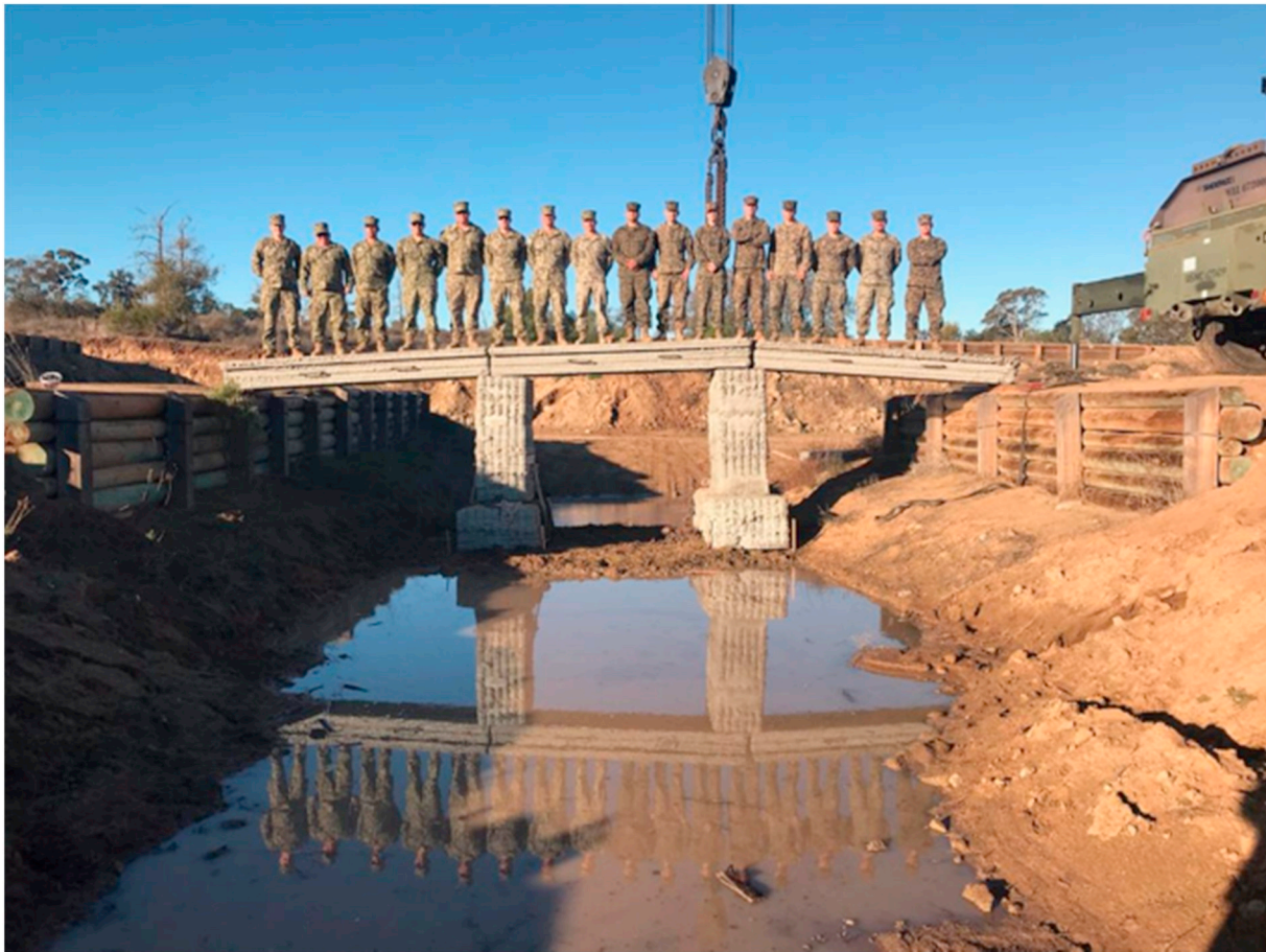
Fig. 6. 3-D printed bridge by the 1st Marine Logistics Group of the U.S. Marine Corps, in December 2018 (photo courtesy: Dr. Michael Case, U.S. Army Corps of Engineers).
