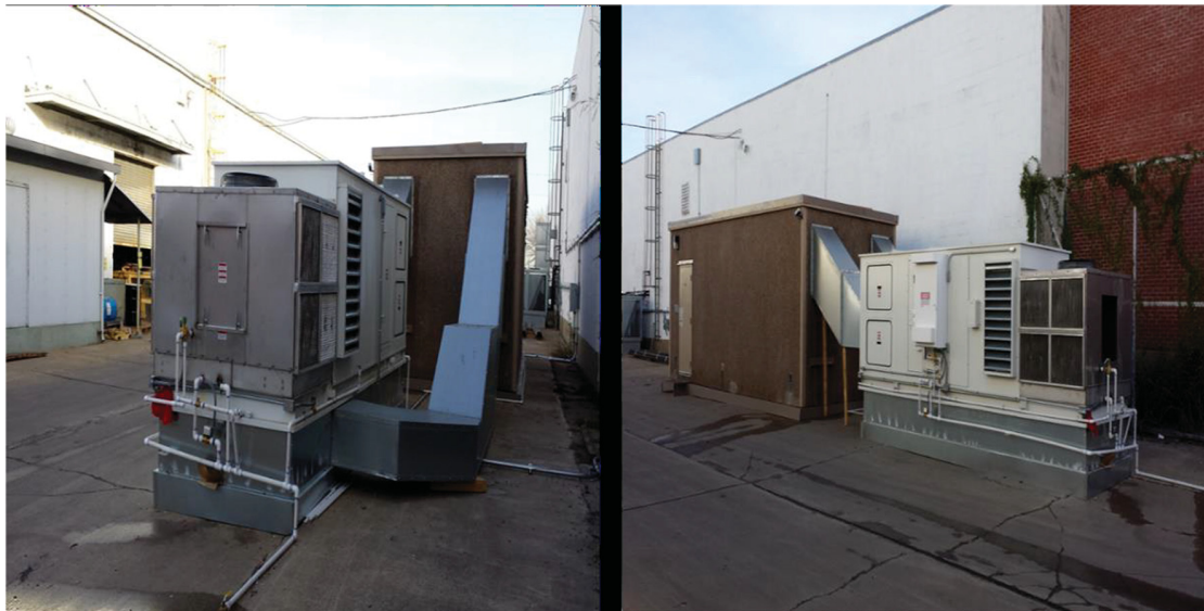
Fig. 3 Cooling unit and IT pod of the modular data center
