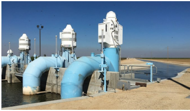
Fig. 6. (Color) Water banking facilities at the Semitropic Water Storage District allow water storage in Kern County, CA, and reverse flow of stored water back to the California Aqueduct. (Image by authors.)
