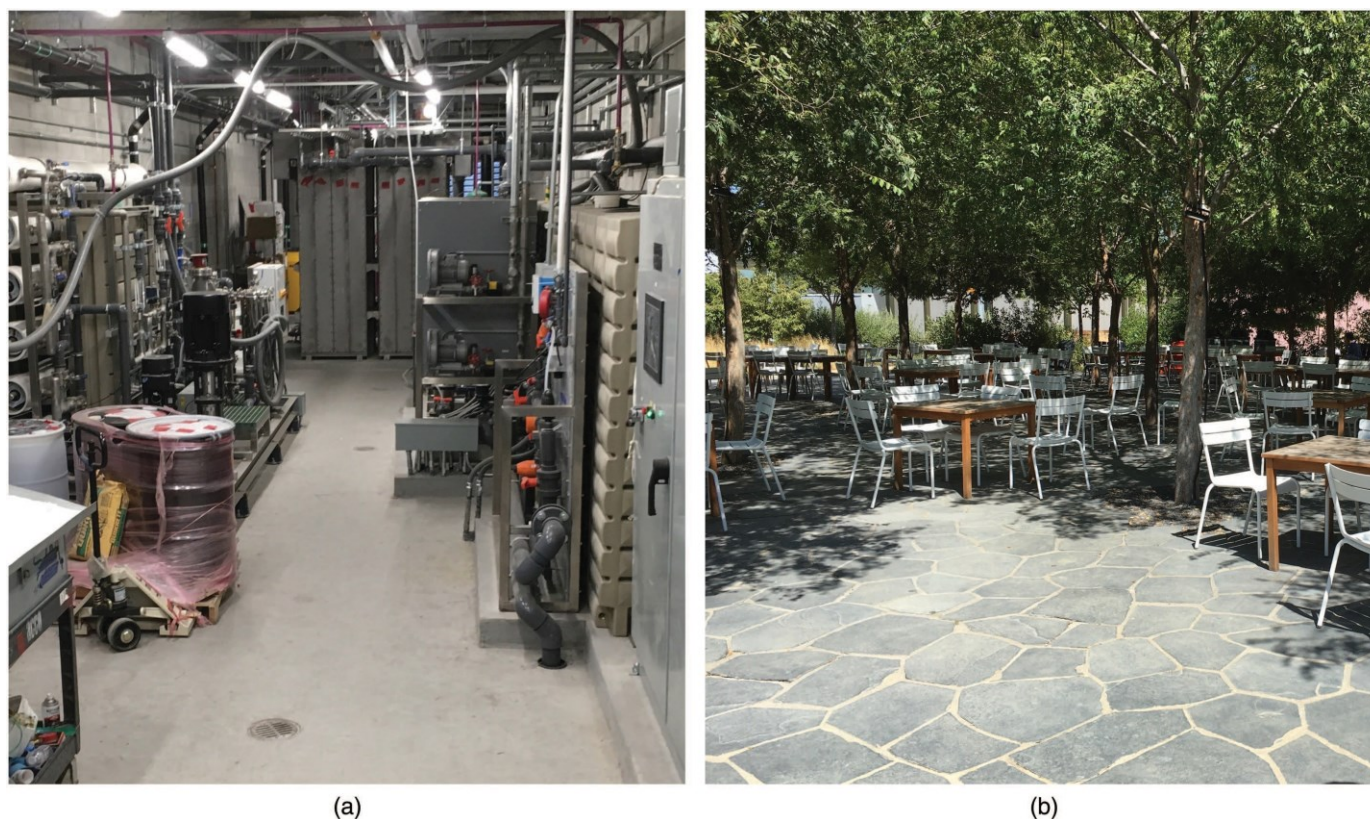
Fig. 4. (Color) Facebook's nonpotable reuse system (a) comprises microscreening, membrane bioreactors, reverse osmosis, and UV disinfection with chloramine and mineral adjustment; (b) The system is designed for 61,000 m 3 /yr (16 million gal./year) for irrigation of 5.3 ha (13 acres) of rooftop gardens and gathering spaces. This is an example of distributed water reuse, which is gaining popularity at large tech campuses and office buildings in California. (Images by authors.)
