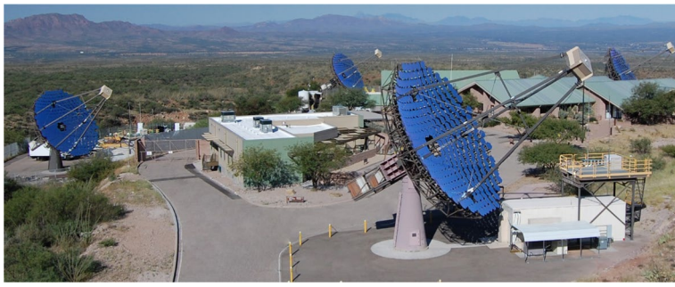
Fig. 1 | The VERITAS array. Left, Photograph of VERITAS located at the Fred Lawrence Whipple Observatory located in Amado, Arizona, USA. The array consists of four 12-m diameter telescopes, T1 (front centre), T2 (leftmost), T3 (rightmost) and T4 (back centre). The right plot shows a top-down view of the array with each of the radial telescope separations.
