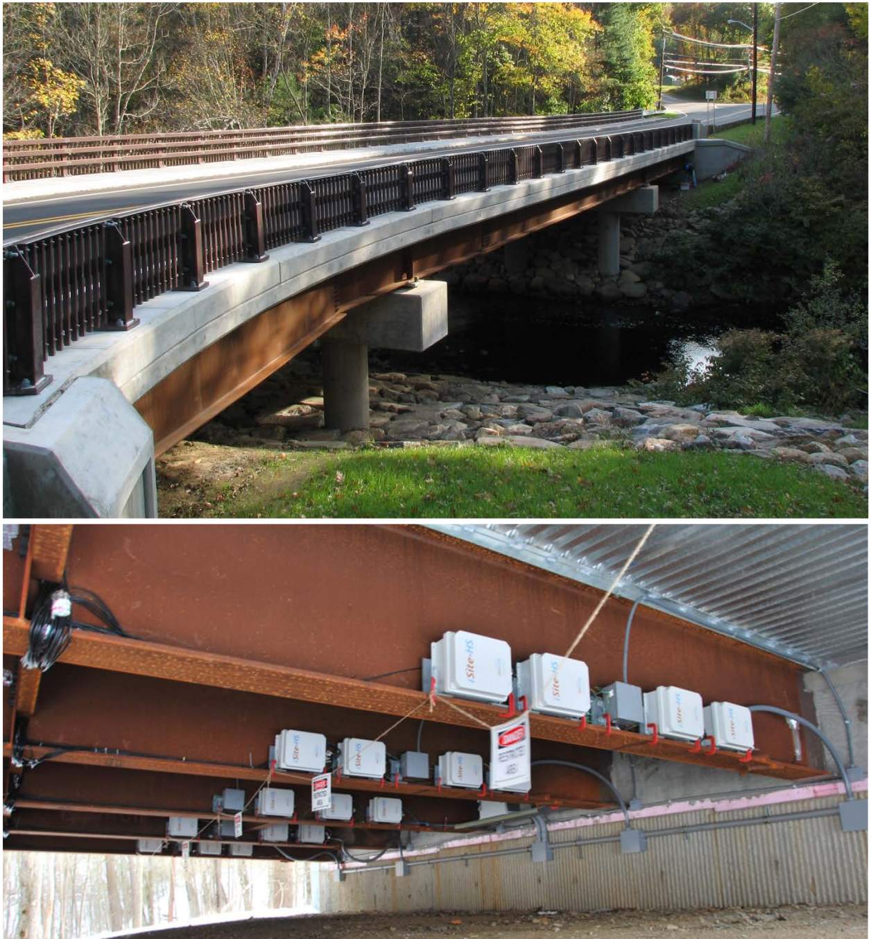
Figure 1. Above: Powder Mill Bridge in Barre, Massachusetts, USA; Below: Data acquisition system underneath the bridge by Geocomp
