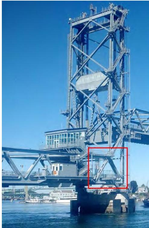
**FIG. 14. Picture of the south tower and fixed truss with the truss-tower connection outlined showing gusset plates tying the two together**
