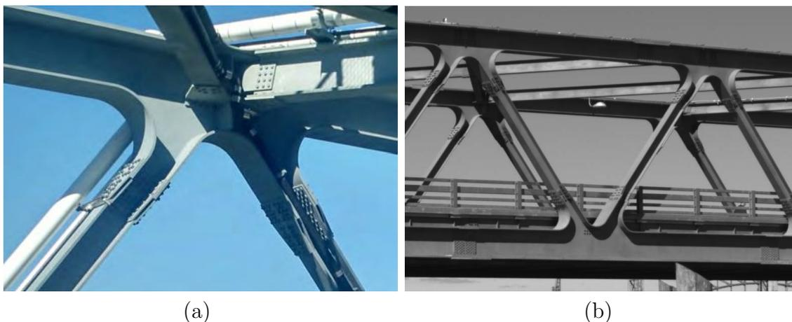
**FIG. 13. Pictures of the special connections on the bridge with a monolithic joint and the gusset plates moved onto the elements with pictures from the (a) bridge interior showing diagonal supports between the trusses and (b) bridge exterior**
