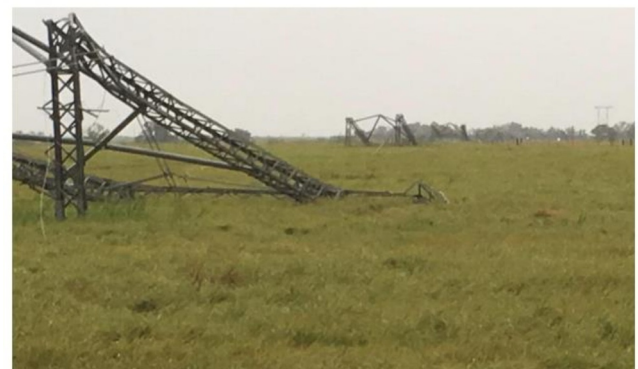
Fig. 1. Reported 345 kV line structure down during hurricane Harvey [23].
