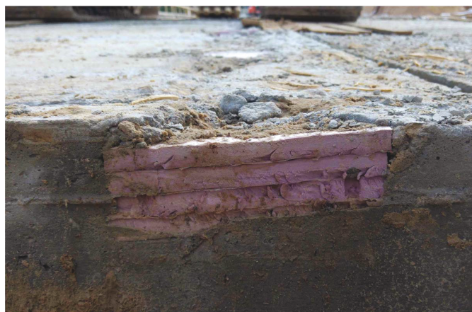
Fig. 5. Shear key blockout. (Image by Thomas Cadenazzi.)
