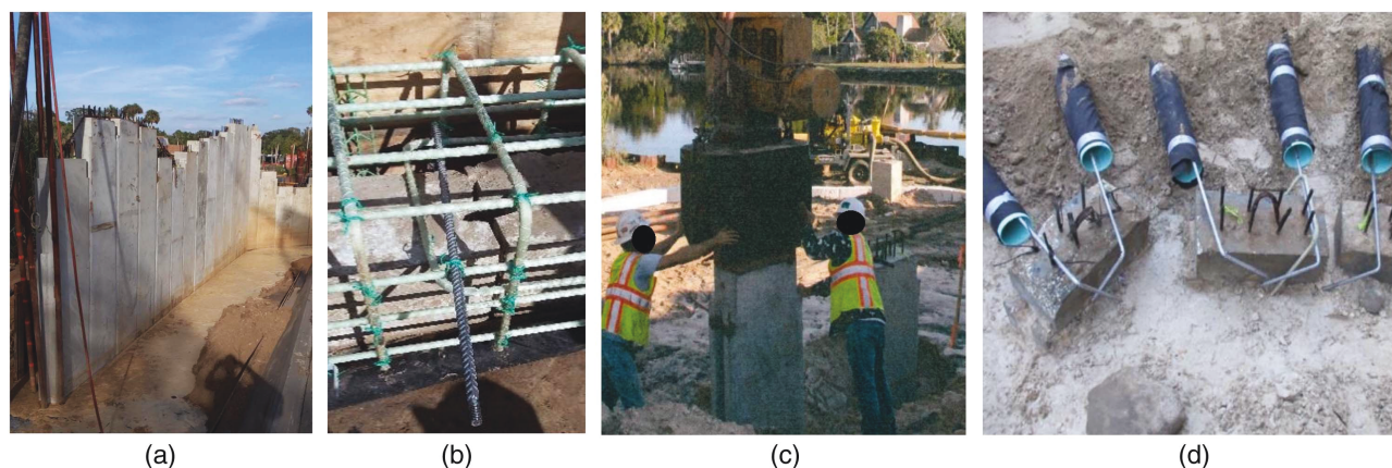
Fig. 14. (a) Cantilevered sheet pile wall; (b) anchored sheet pile wall through SS rods; (c) deadman anchor installation; and (d) SS rods anchored to deadmen prior to casting of the deadmen cap. (Images by Thomas Cadenazzi.)
