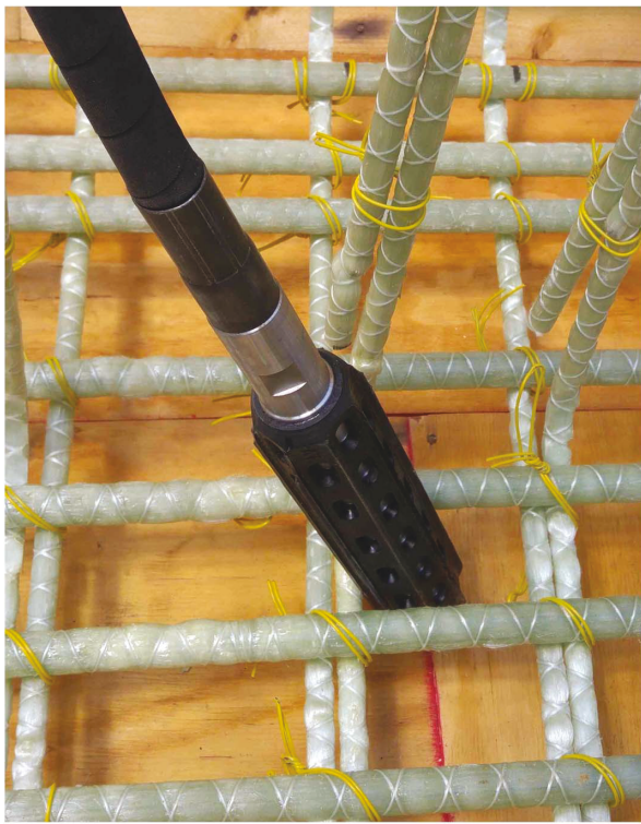
Fig. 3. Rubber-tipped vibrator. (Image by Thomas Cadenazzi.)
