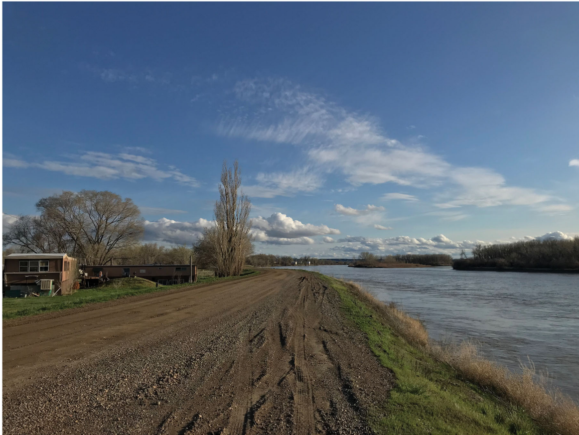
Figure 3. Miles City levee just downstream from the Tongue and Yellowstone Rivers' confluence. The view is looking upstream. Note the proximity of the levee to the Yellowstone River, the gravel roadbed on top of the levee, the tree growing out of the levee's side, and the structures near the levee. Source: Kirsten Bergmann.
