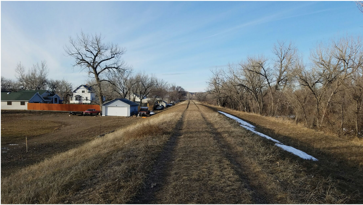
Figure 5. West Glendive levee near the western terminus of the Towne Street Bridge. The view is looking downstream. Note that no vegetation is growing on the levee and that the river is not visible. Source: Elizabeth A. Shanahan.
