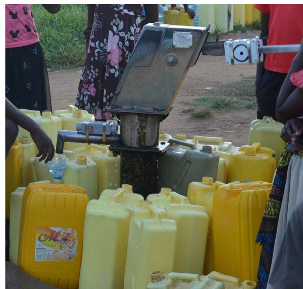
Fig. 5 Pump site in northern Uganda with the sensor mounted to the pump handle
