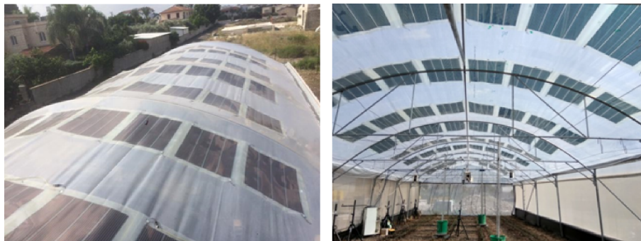
Fig. 1. OPV panel arrangement on the tunnel roof. Photos were taken from outside (left) and inside the tunnel (right) respectively.
