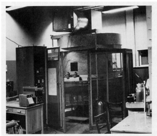
Fig. 21: Improved Ward-Type simulator used by Leslie (1977). © American Meteorological Society. Used with permission. [107].
