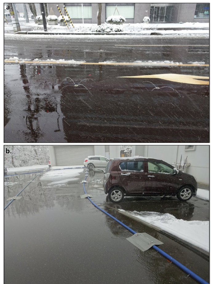
FIG. 8. Snow melting and removal using (a) road sprinklers in Nagano and (b) water tubes at the Snow and Ice Research Center in Nagaoka.
