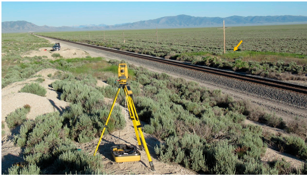
Figure 4. Site where the laser total station was installed for surveying Transects A and B. The vertical survey point LQ0282, to which the total station survey was referenced, is located 65 m away on the other side of the railroad line (orange arrow).
