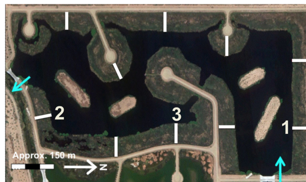
Fig. 1 Aerial image of the Tres Rios Constructed Treatment Wetland in Phoenix, AZ. Arrows represent the inflow and outflow, and numbers and white lines show the location of the marsh transects where water quality samples were taken
