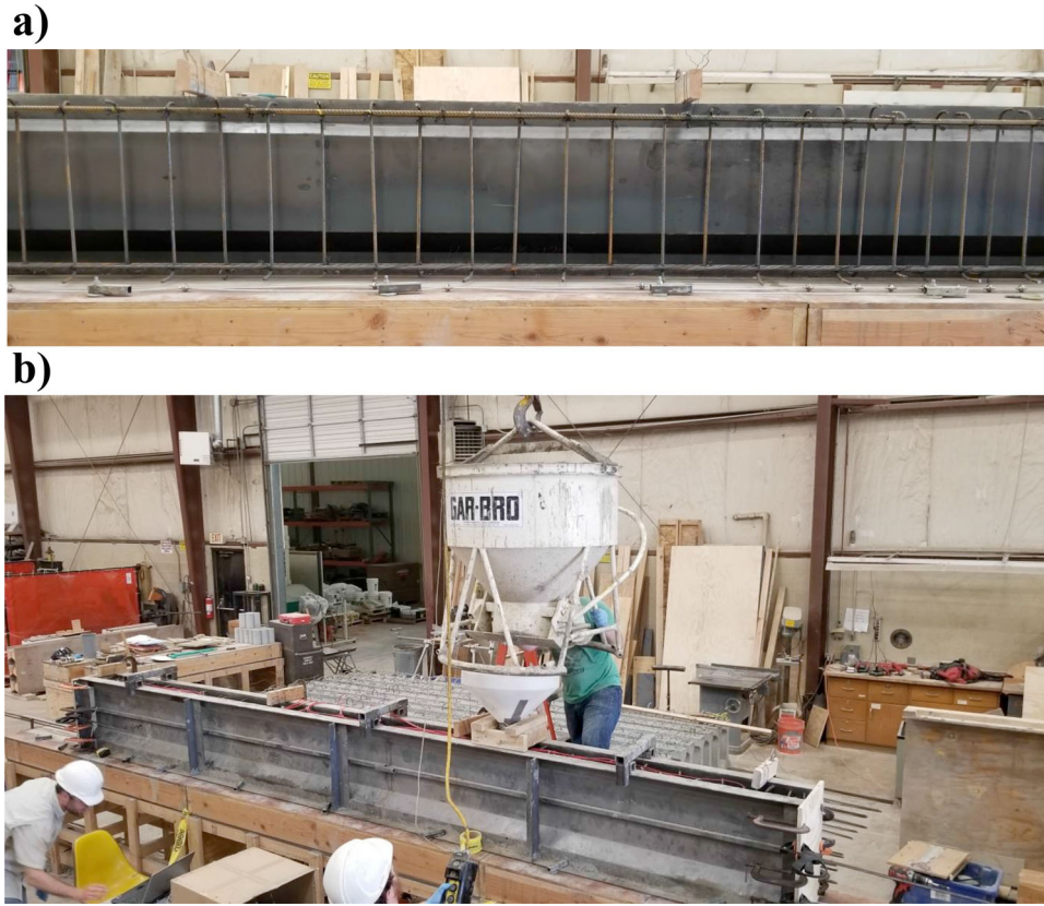
Figure 5. View of (a) beam reinforcement before casting and (b) beam during construction.
