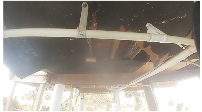
Fig. 8. Floor underside cladding damage on the southeastern edge of Building 225. (Photo credit: Josh Hunt, University of Alabama.)
