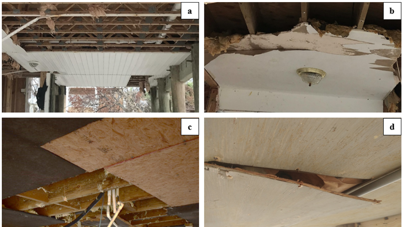
Fig. 4. Types of floor underside cladding and damage observed after Hurricane Michael; (a) vinyl with fastener failure, (b) hardboard with panel failure, and (c, d) wood structural panels with fastener failure. (Photo credits: (a, b) Elaina Sutley, University of Kansas, (c) Josh Hunt, University of Alabama, (d) Jae Kim, University of Kansas.)
