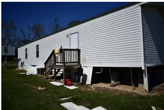
Fig. 2. Manufactured home situated on concrete block footers with damaged and partially-removed skirting, damaged in 2018 Hurricane Michael. (Photo credit: Josh Hunt, University of Alabama.)
