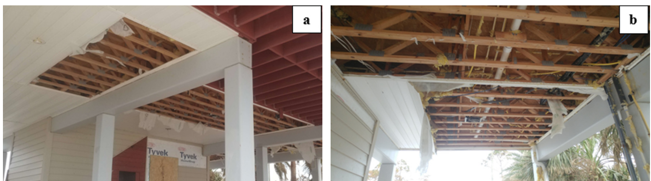
Fig. 6. Examples of large sections of cladding panel loss on the floor underside. (Photo credit: Jae Kim, University of Kansas.)
