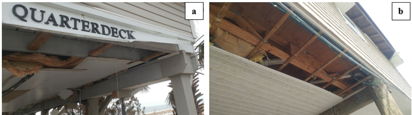
Fig. 5. Examples of edge and corner floor underside cladding damage. (Photo credit: Jae Kim, University of Kansas.)
