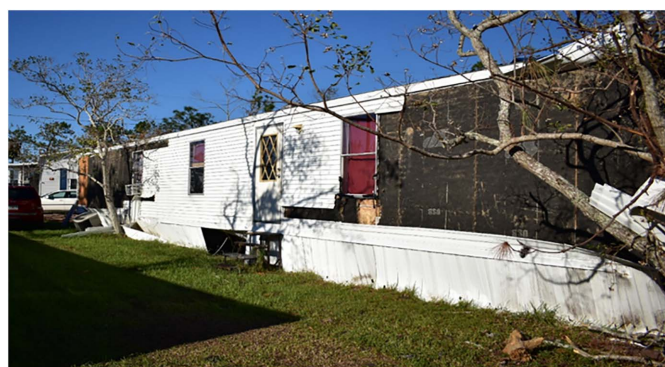
Fig. 5. Damage state 3 classification example. (Image by authors.)
