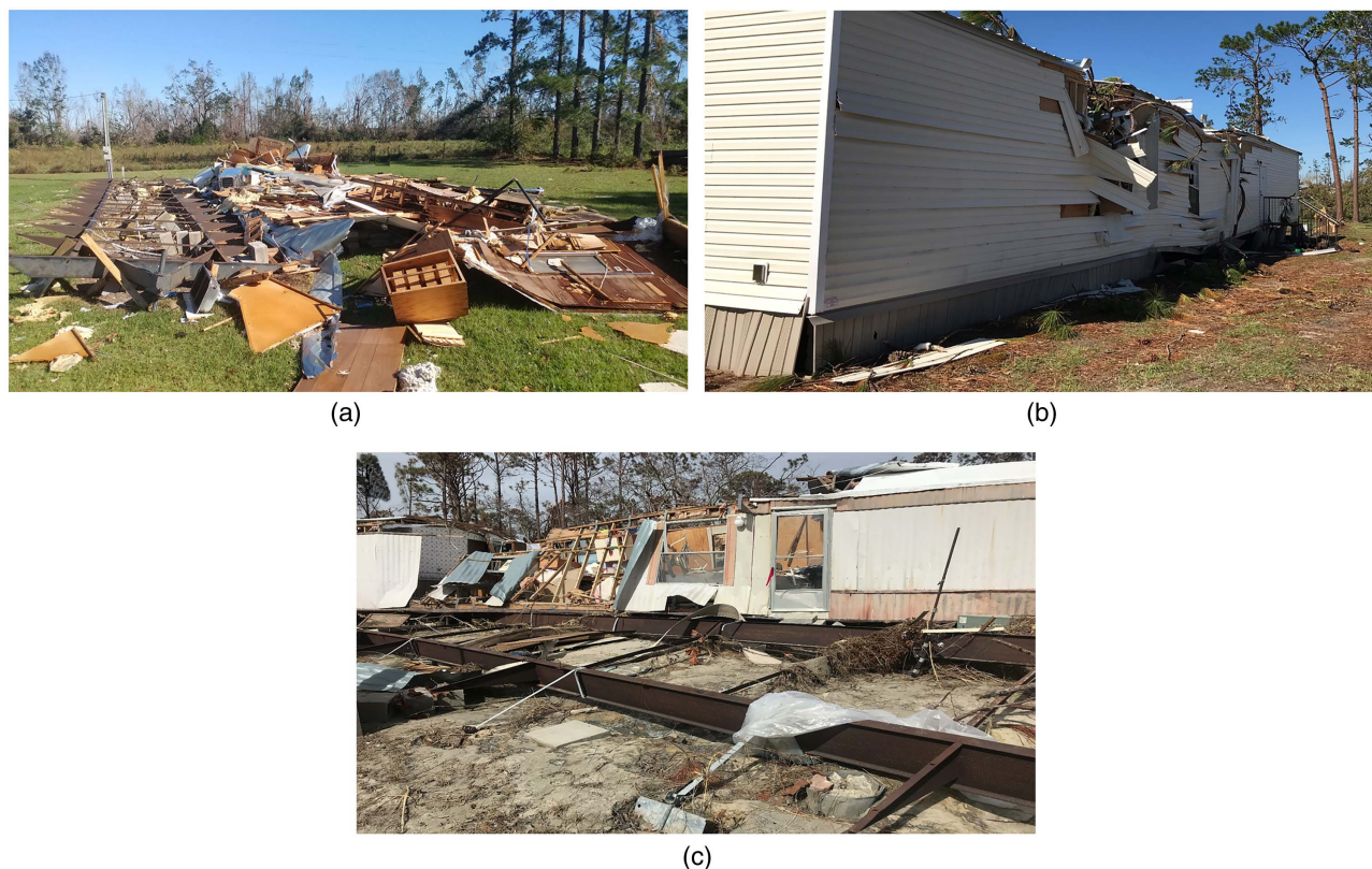
Fig. 6. Damage state 4 classification example: (a) exploded home; (b) tree-destroyed home; and (c) surge-dislocated and partially collapsed home. (Images by authors.)
