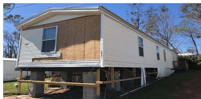
Fig. 4. Damage state 2 classification example. (Image by authors.)
