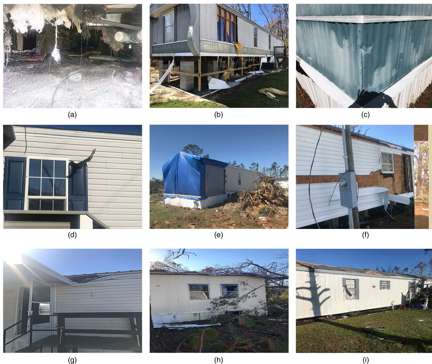
Fig. 11. Damage to trailer: (a) floor underside damage; (b) skirting and siding loss; (c) siding indentation; (d) debris missile; (e) tarping covering portions of the roof and wall structure; (f) siding and skirting removed with a full-height hole in the wall structure; (g) hole in the roof; (h) tree fall onto roof; and (i) roof shingle loss. (Images by authors.)
