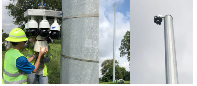
Figure 6. Multi-camera mount is raised onto 110 ft pole.
