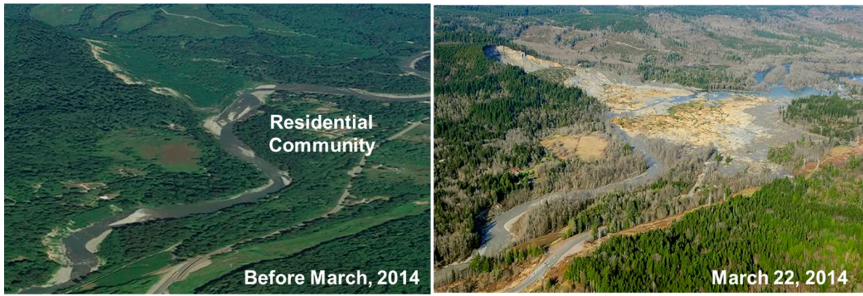
Figure 1. Aerial photographs of Oso slope before and after the March 2014 failure.
