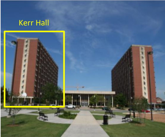
Figure 1. Kerr Hall (investigated building)
