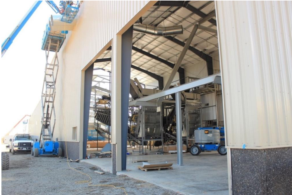
Figure 5: Smaller hop picker being built to allow for simultaneous harvest of boutique, test, or uncommon hop varieties without interrupting harvest of larger-acreage varieties (such as Citra™, Simcoe™, etc.). These hop pickers clean and pick hops from bines which are cut in the field and brought to these large warehouse settings for picking, kilning, curing, and baling.
