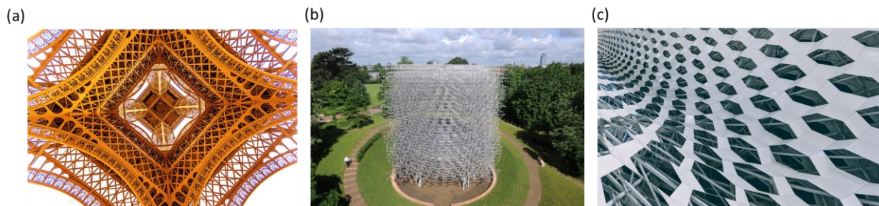
Figure 2 – (a) Upward view of the Eiffel Tower in Paris, showing hierarchical structure of 18,000 iron parts (mostly struts) connected with 250 million rivets. 59 (b) The Hive , installed in London’s Kew Gardens in 2016, simulates a living beehive. Its lattice, 17 m in height, comprises 170,000 aluminum struts and connectors. 60 (c) A view inside the Bao'an airport at Shenzhen, with a 450,000 steel member structure allowing for high earthquake loads, with cross bracings providing high stiffness 61 (photo courtesy: Prof. J. Huang, Northwestern University, IL, USA).
