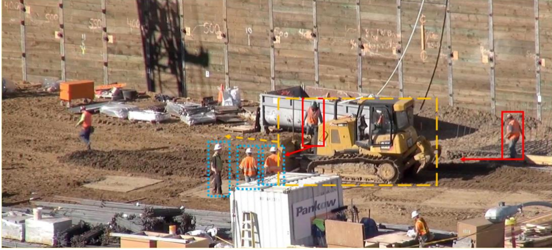
Figure 2 Construction scenario with potential struck-by hazard
