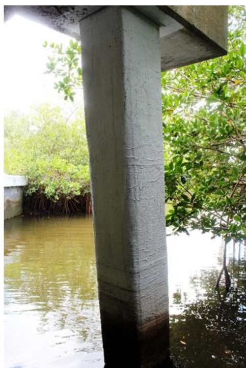
Figure 3. Example of contact-critical application of EB FRP: FRP-confined column in a Bridge in Florida, USA (note: FRP wrap is painted).
