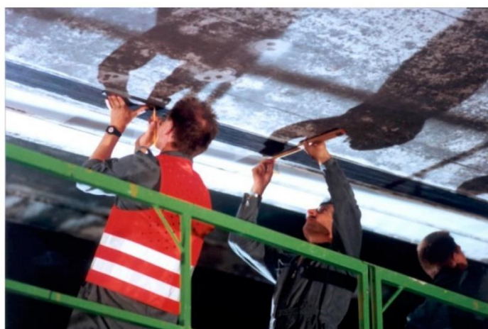
Figure 1. Application of externally bonded (EB) fiber-reinforced polymer (FRP) strips on a bridge headscarp in Switzerland in 1991, what is believed to be the first application of EB FRP in the world (reproduced from [4]).
