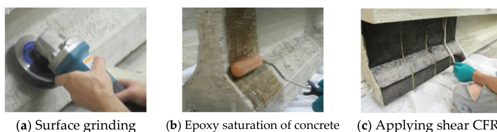
Figure 4. (a–c) EB FRP installation (reprinted from [24]).
