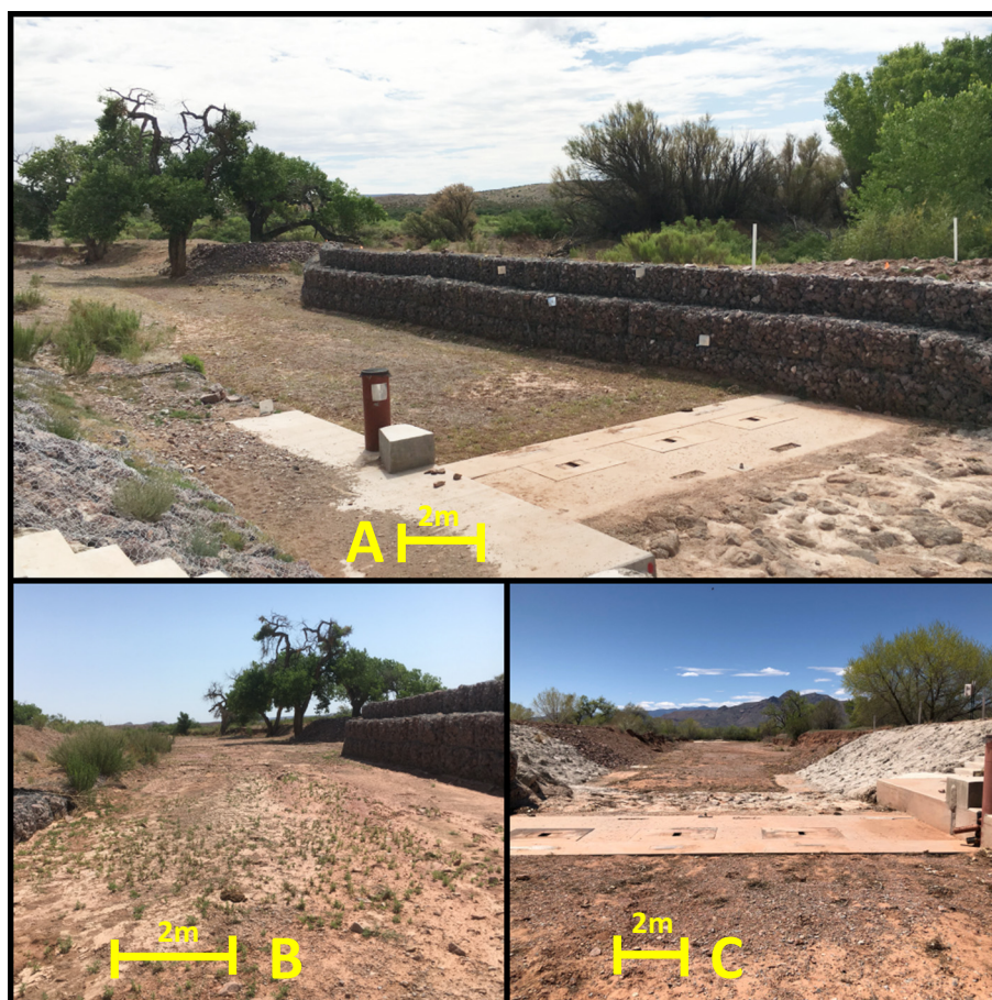
Fig. 3. Photos of constructed Pinos site in oblique view (A), looking upstream (B) and looking downstream (C).
