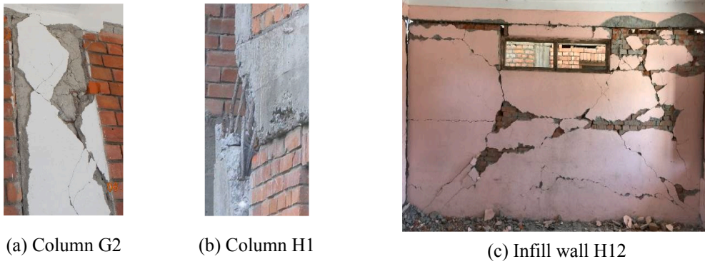
Fig. 2. Observed damages in the first story of the building.
