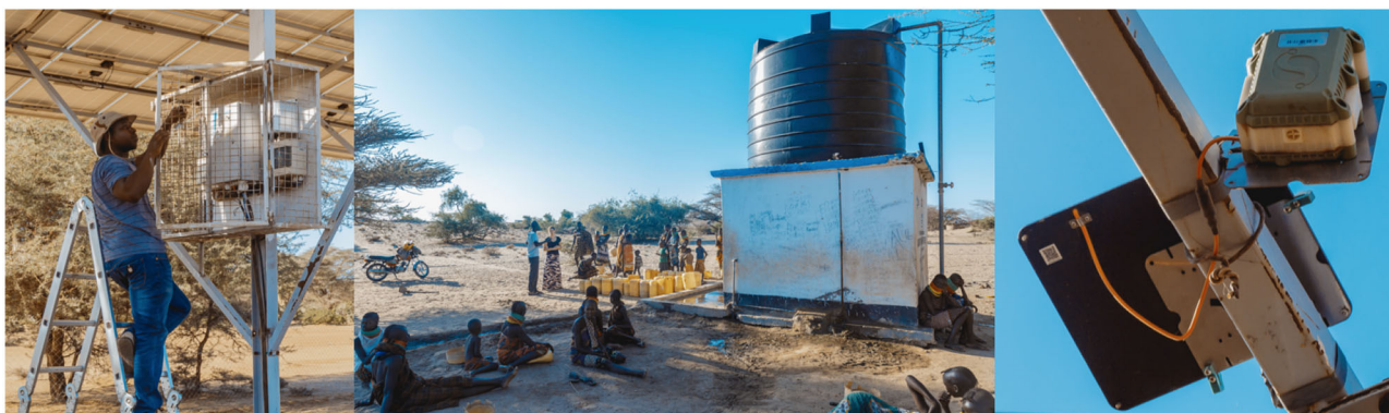
FIGURE 2 | A typical groundwater borehole in Turkana, Kenya (center). Electrical monitoring sensors are installed at the pump controller (left), and wireless transmit data to a self-powered satellite or cellular transmitter ( www.sweetsensors.com ).
