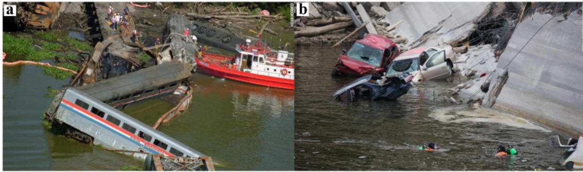
Fig. 1. Some of the serious recent bridge accidents in the US: (a) A collapsed railroad bridge in Alabama that resulted in around 47 deaths. (b) Collapsed bridge that connected Point Pleasant, West Virginia with Gallipolis, Ohio [1].
