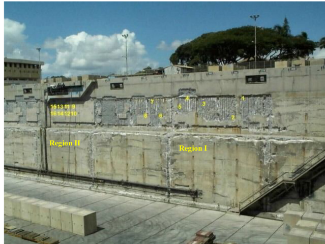
Fig. 1. Dry-dock fascia photograph taken at the time of the repair (2001) also showing approximate locations of cores taken in 2019.
