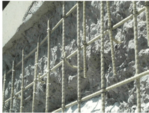
Fig. 3. Doweled GFRP reinforcement grid in the fascia of the dry-dock (Region II).
