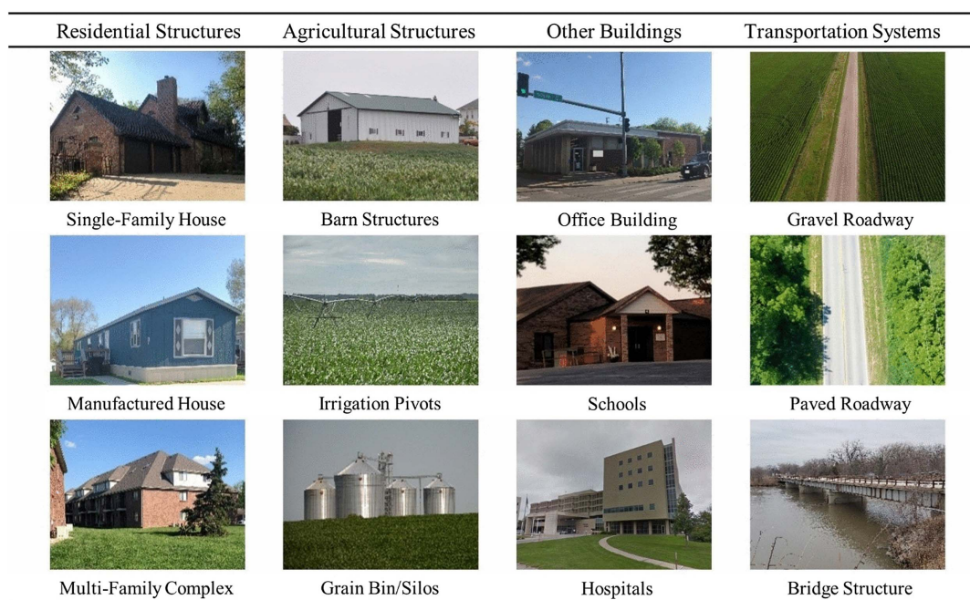
Fig. 2. General classifications for structures in the digital reconnaissance, excluding the other , lifeline , and unspecified categories. (Images by authors.)
