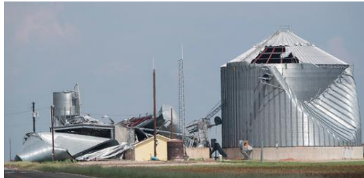
Figure 2. Three collapsed and severely damaged grain silos following Hurricane Harvey in Refugio, TX (photo courtesy of US Department of Agriculture: https://www.flickr.com/photos/usdagov/36508165554 ).
