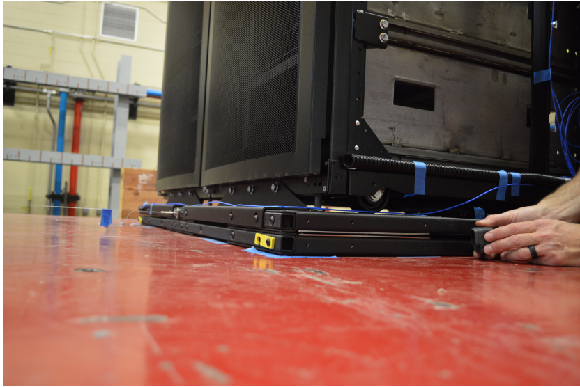
Figure 3.13: Reduced platform clearance of isolation system.
